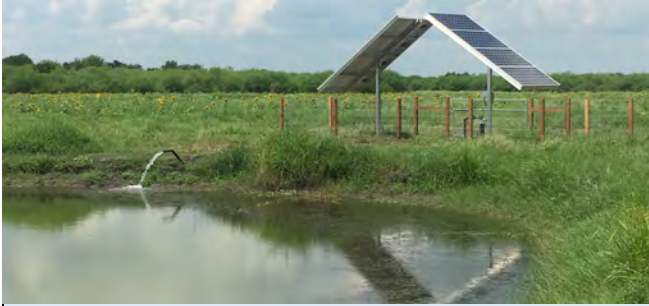
Solar wells can be used to maintain flooding in small wetlands, especially during drought.
